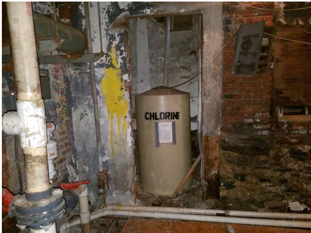
Photograph No. 20: Photograph of choline AST located within the eastern potions of the subject building basement.
