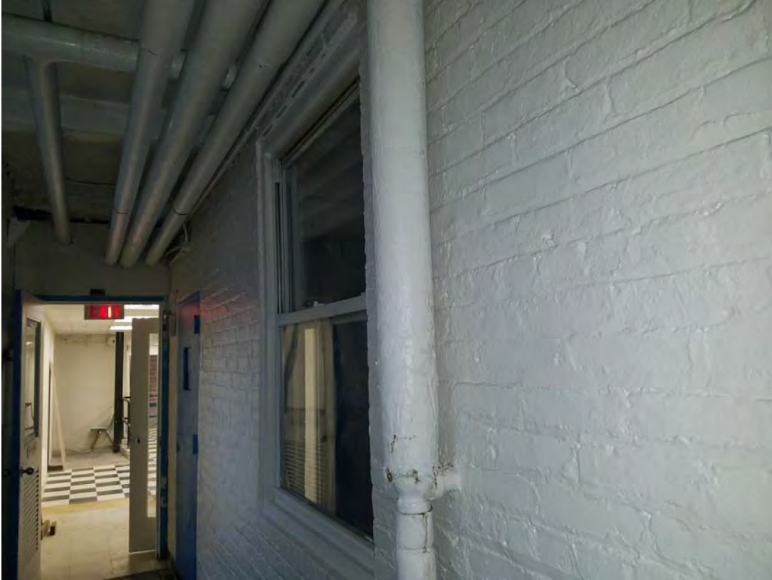
Photograph No. 23: Representative photograph of the suspect ACM pipe insulation located throughout the subject building.
